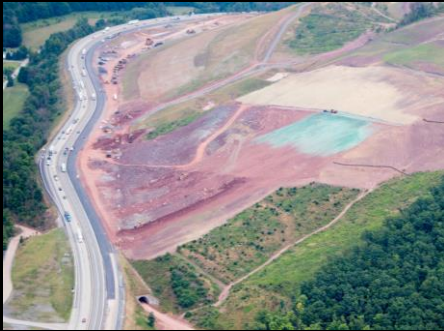
Slide Repair & Construction Management
