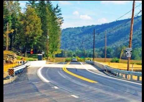
Roadway Construction Inspection
