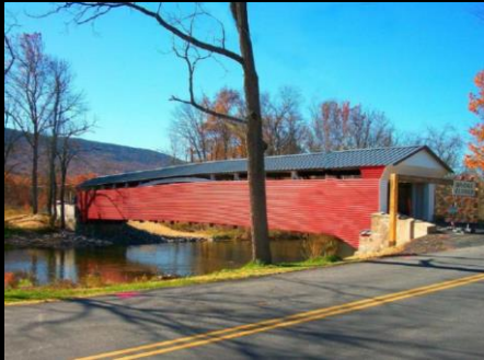
Bridge/Tunnel Construction Inspection
