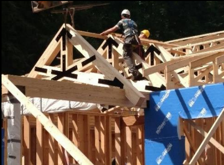
Open-End Construction Inspection
