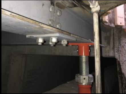
Construction Shoring & Falsework
